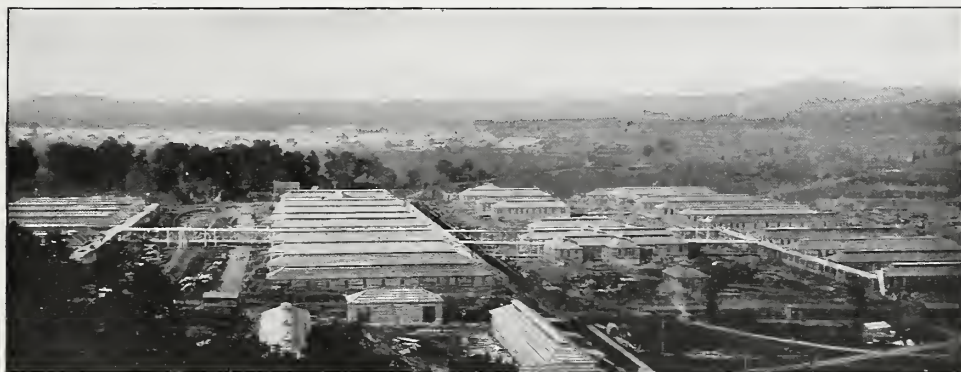
FIG. 197.—View of Base Hospital, Camp Sherman, Chillicothe, Ohio.
